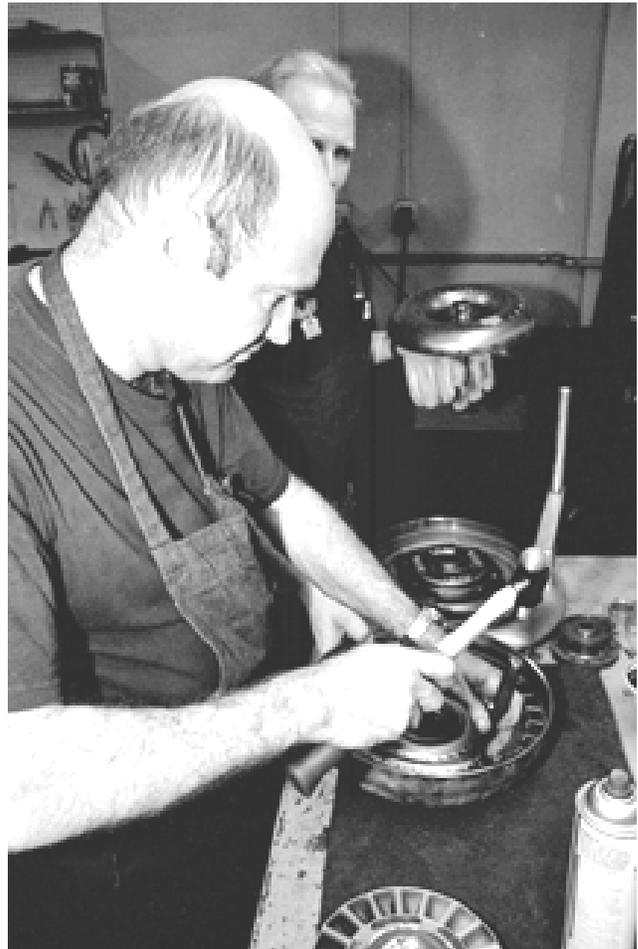
*In addition to altering blade angle as required, William deftly uses a punch and hammer to tighten every fin prior to welding. More important small details.*
