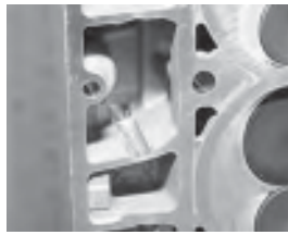
Cylinder heads feature pushrod clearance reliefs.
